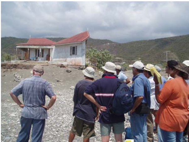
Above: Group observing the damage caused by hurricane Ivan at Copacabana
